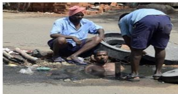
Fig 1. Drainage with manual workers
